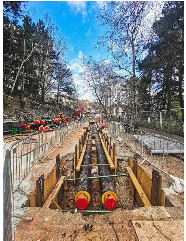
Photo credit Vital Energi
